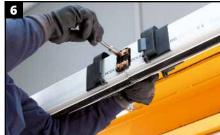
Cover the connection, sliding the **joints RG02 (both halves)** until completely closed **(click)** using the pressure tabs (Photos 7, 8 and 9). In outdoor lines we recommend using screws at the lower of the joint.
