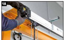
Install the corresponding towing arm RG06 or RG08 (Photo 19), or RG06POL (Photo 20), aligning it with the central axis of the conductor bars, and slightly lower than the collector trolley. It is very important that the pulling is parallel to the axis of the line. The collector trolley cable should be installed forming sufficient loop, to not cause any torsion of the trolley (Photos 19 and 20)
